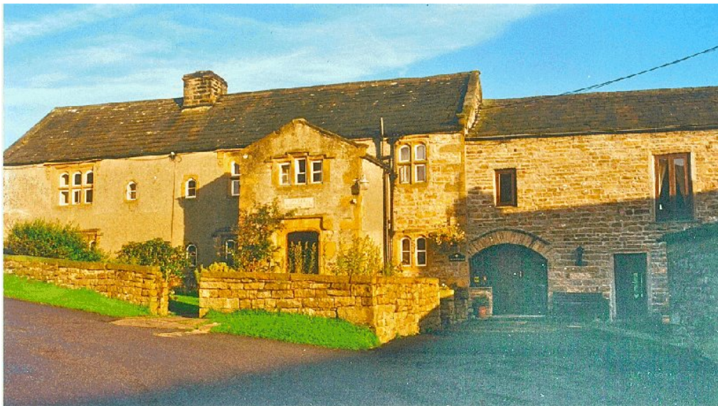
Figure 4 - Oxnop Hall as it is today, with the new large porch which was reassembled onto the front of the main house probably in about 1685. The old west wall had collapsed probably after 1764, (its foundations below ground level are still present) the new replacement west wall being relocated eastwards, shortening the house by some 20 feet. The eastern side carriage house wing has had a second story added in later times.
